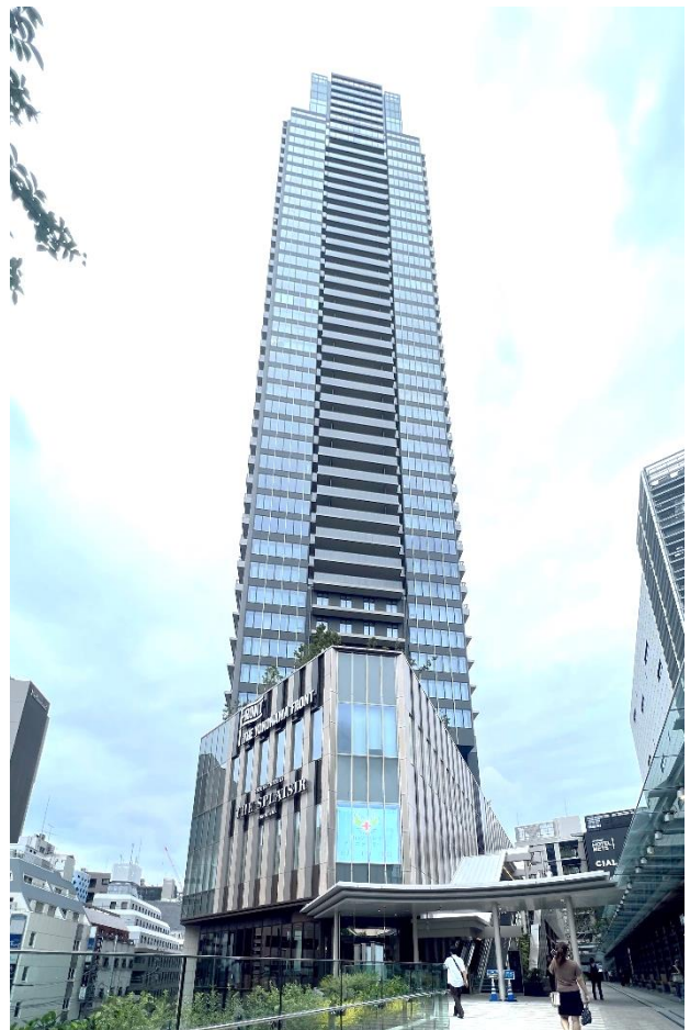
THE YOKOHAMA FRONT TOWER 完工現況(本基金會攝)
